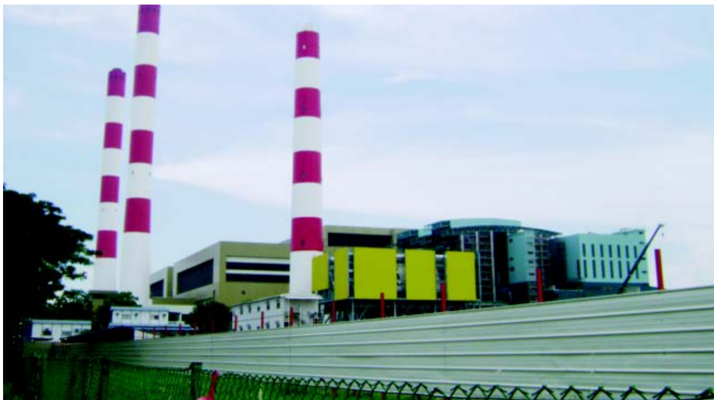
Large scale MSW plant in Singapore
